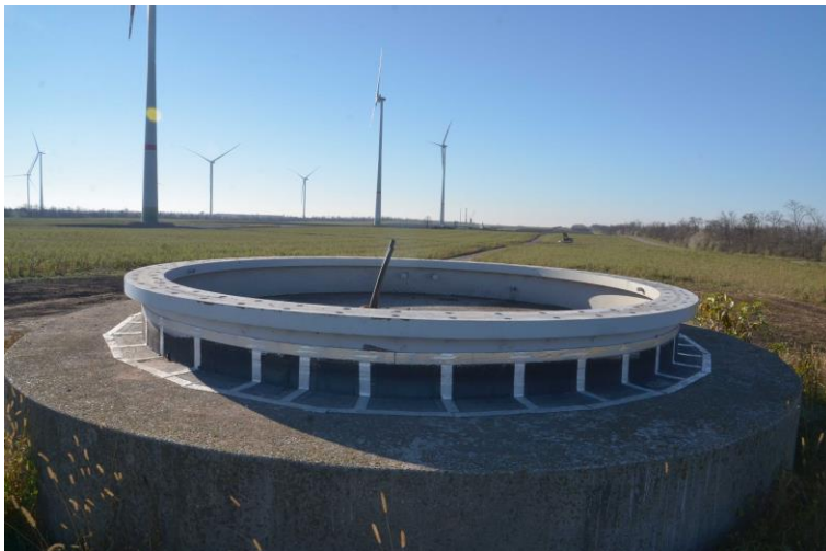
Photo 07-05: Dismantling of existing wind turbines on the Parndorf Plain, then repowering
