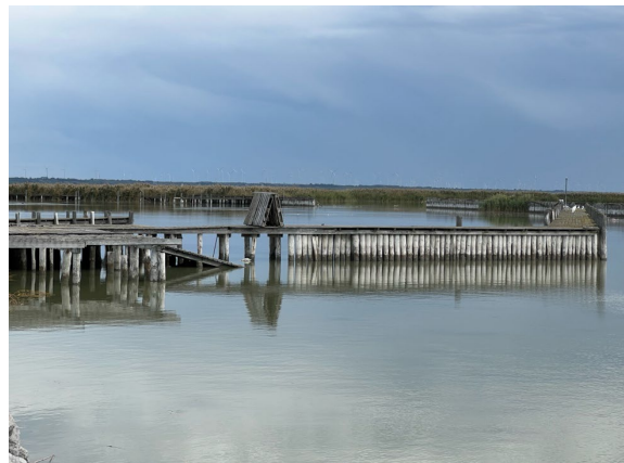
The old yacht harbour at Breitenbrunn Resort which will be rehabilitated as natural area
