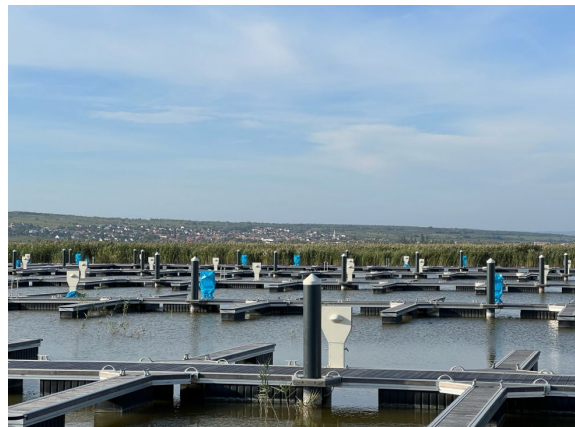
Northernmost harbour near completion
