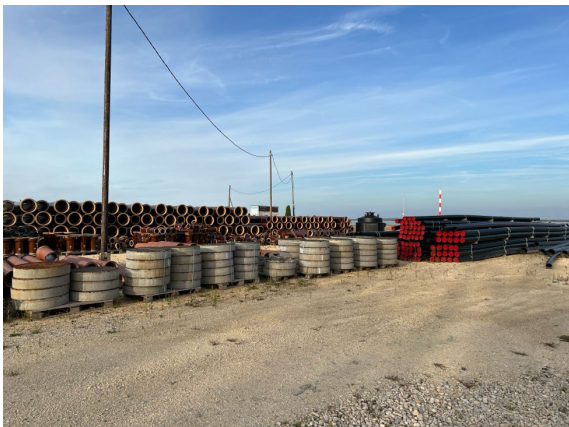
Elements for sub-surface infrastructure on site
