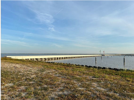
Future beach with concrete infrastructure
