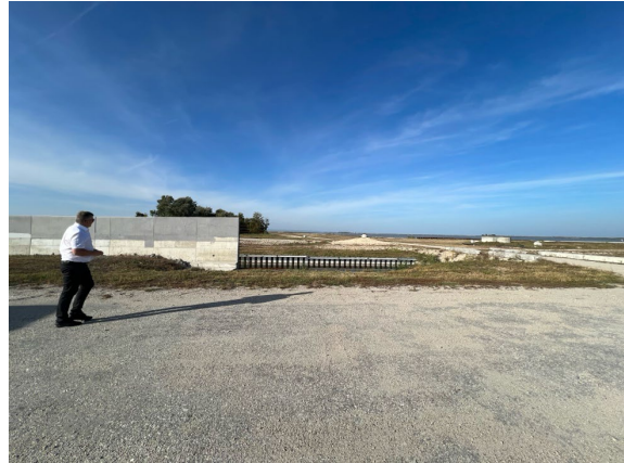
New concrete wall at the entrance to the redevelopment site
