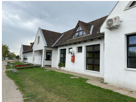
Existing buildings planned to be redeveloped
