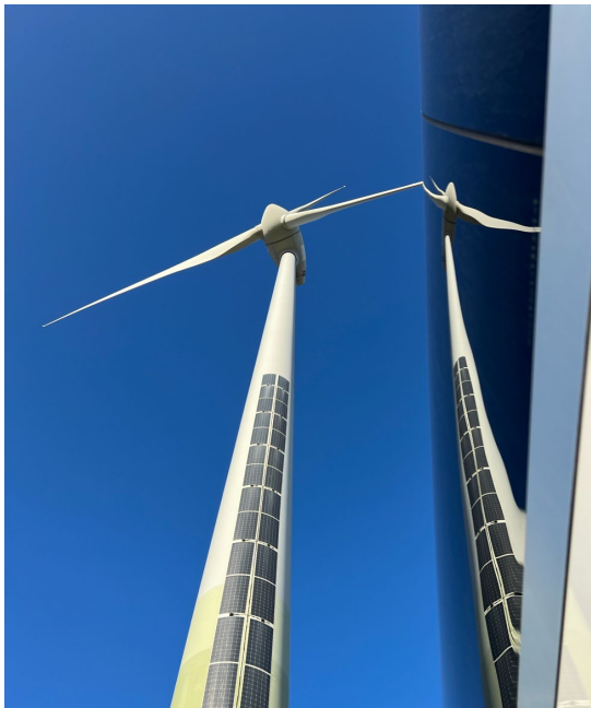
Experimental wind and solar power combination
