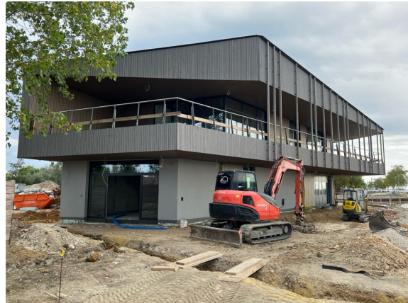
New restaurant building at Breitenbrunn Resort under construction
