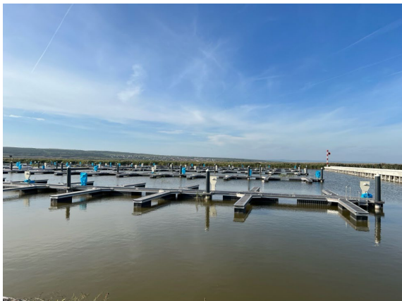
Northernmost harbour near completion
