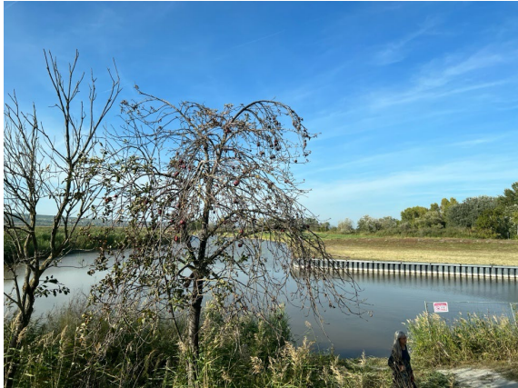
Canal dividing redevelopment site and reed bed separating Sopron-Fertő Lake Resort project site and Fertőrákos
